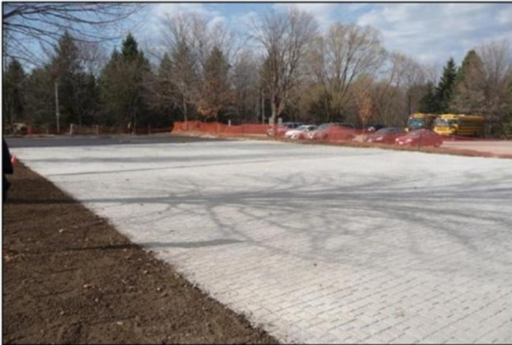
Figure 3.1: Kortright permeable pavements
